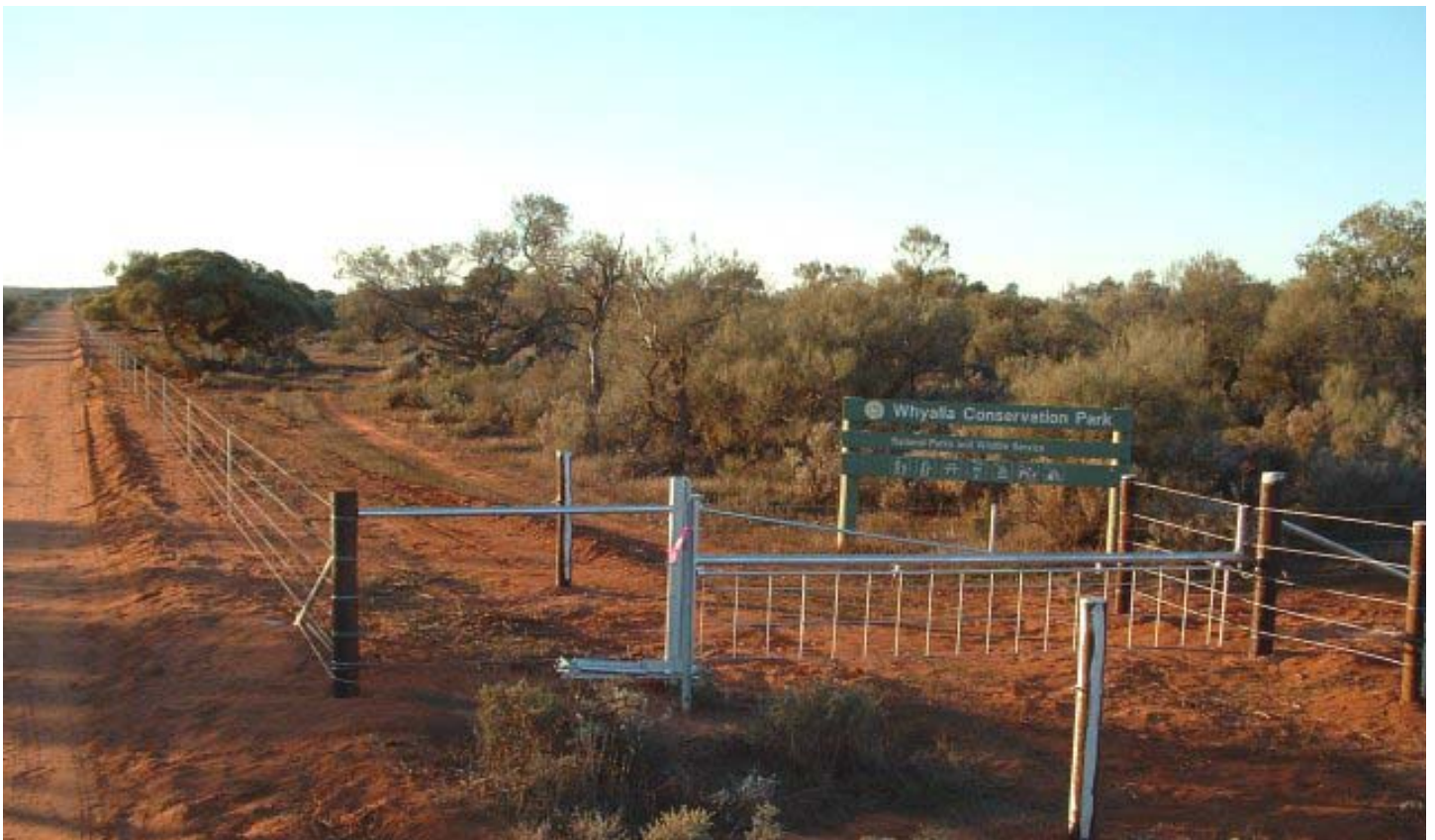
The new fence along the western boundary of the new section of the Park. Shown is the self-closing gate at the south-western corner.
