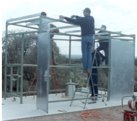
Construction work on the toilet 2000
