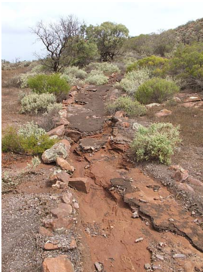
Damage to the section of the walking trail leading up Wild Dog Hill caused by the recent heavy rain.
