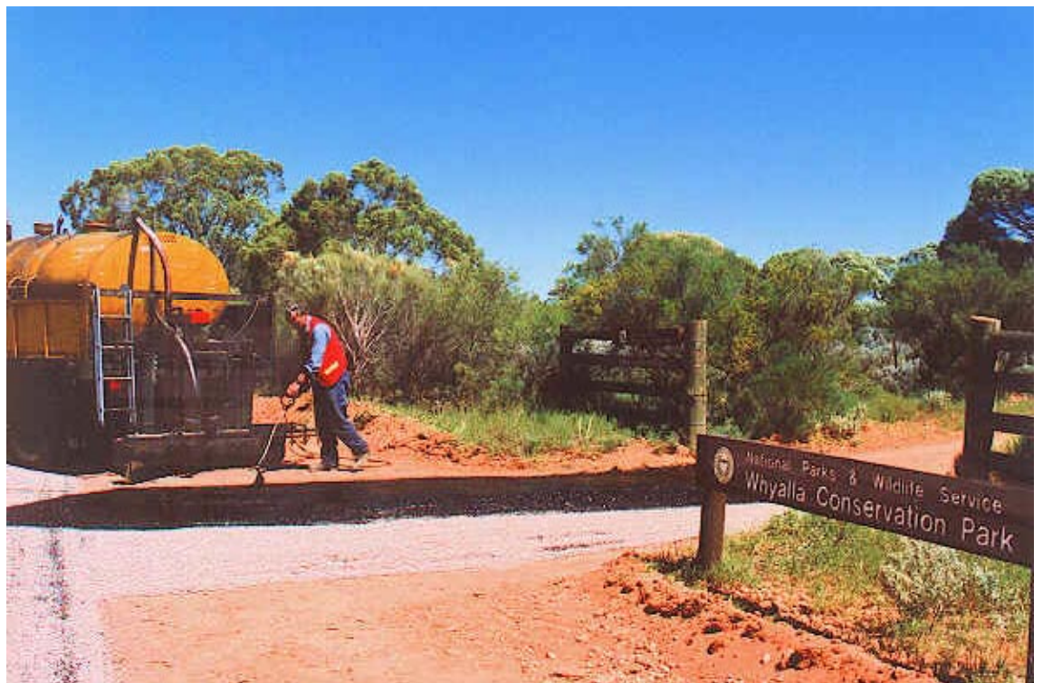
The Department of Road Transport sealing the verges of the highway outside the Park recently.
